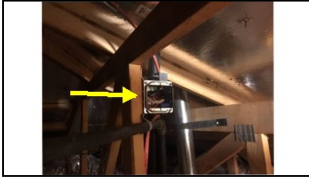
Cover missing at junctions box(es) exposing connections - needs to be serviced
