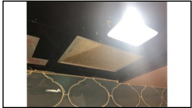
Worn/dirty filters, recommend cleaning or replacing
