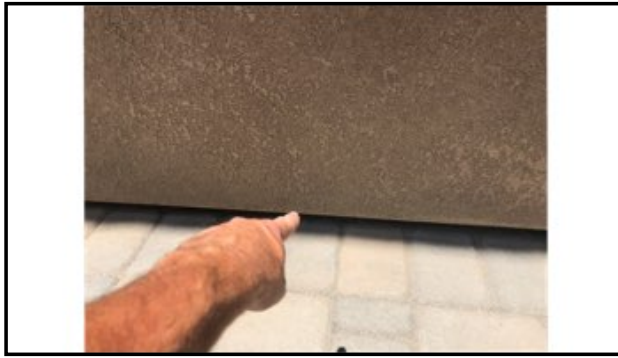
Weep screeds should be minimum 4-inches from grade - needs to be serviced
