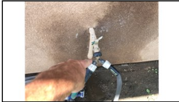
Hose bib at east side of house leaks
