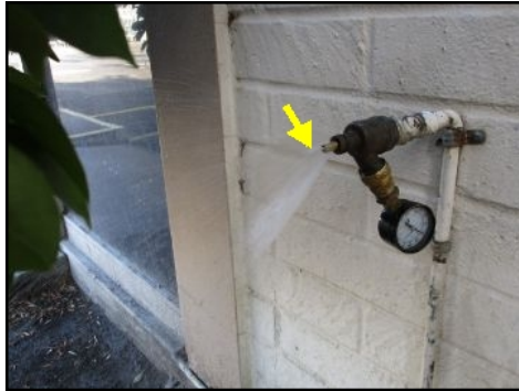
Exterior hose faucet(s) leaked at handle(s) when operated at rear - needs to be serviced
