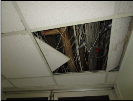
Missing loose panels ,300 - needs to be serviced
