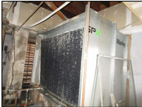
upper roofs chiller/water tower Unit is worn and deteriorated - likely reaching the end of it's life - we recommend that you budget for a replacement and more efficient unit
