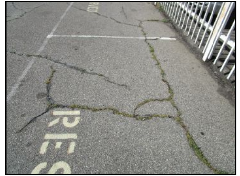
Cracking large at rear parking lot- needs to be serviced
