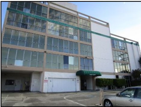
General view of rear
