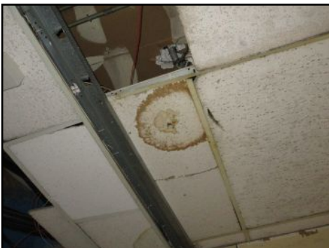
Evidence of leaking from condensation--120
