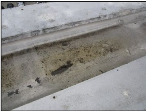
Blistered areas - needs to be serviced
