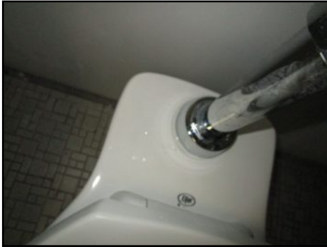
Toilet flush valve was leaking mens 4th floor - needs to be serviced
