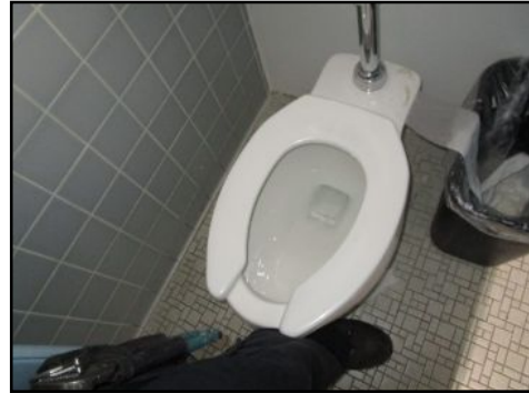
Toilet loose at floor mens 5th floor- needs to be serviced
