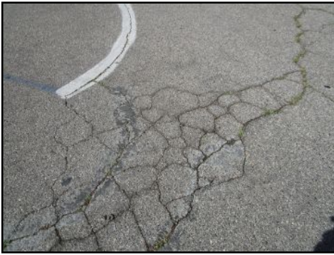
Cracking large at rear parking lot- needs to be serviced
