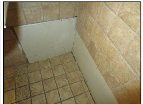
Irregular installation/patching/workmanship & missing tiles 1st & floor mens bath- needs to be serviced
