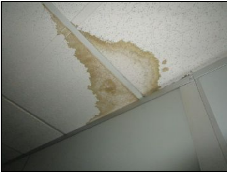
Stains/blistered areas present 200- tested dry with moisture meter
