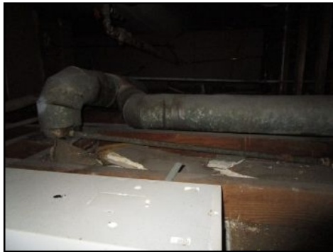
All visible vents appear to be in normal condition where visible - no major visible defects
