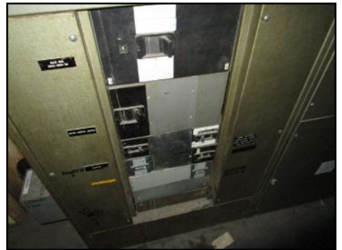
Loose/worn breakers - typical for age
