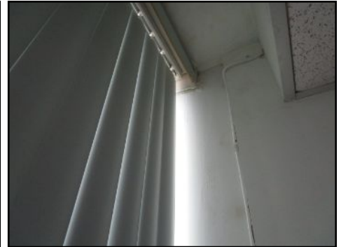
evidence leaking windows south side-2nd floor- needs to be serviced
