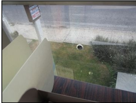
Hole in glass 2nd floor north side - needs to be serviced
