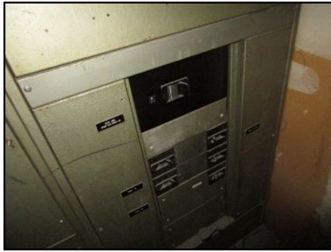
Loose/worn breakers - typical for age
