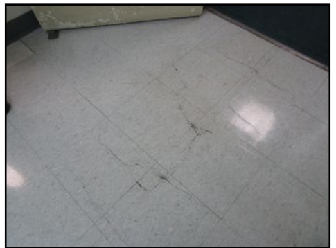
Cracked areas 400- needs to be serviced
