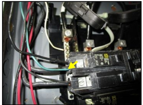
Double tapped/lugged breakers present are a sign of any overloaded panel 1st floor closet by womens bath – recommend licensed electrician for evaluation
