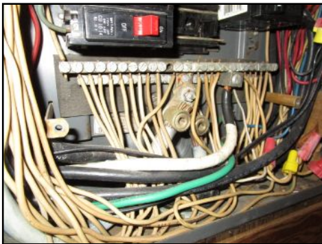
Wiring type: copper
