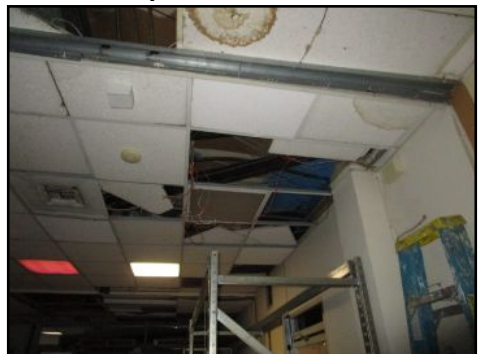
Stains/blistered areas present 1st floor 120- tested dry with moisture meter
