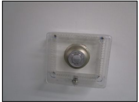
Worn/older model - recommend upgrading
