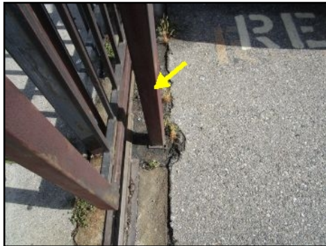
Support posts loose/deteriorated/leaning at west gate parking lot - needs to be serviced
