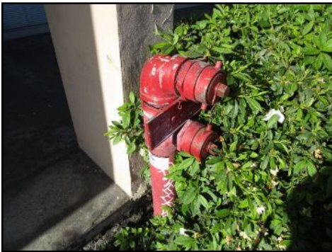
Note: Fire hose present in halls are not inspected
