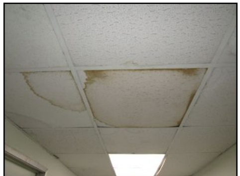
Evidence of leaking from condensation- 2nd floors halls
