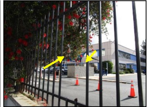
Damaged fencing east side- needs to be serviced
