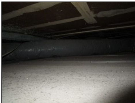
Older/worn ducts present - recommend routine maintenance and cleaning to extend the life of the existing ducts
