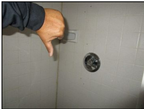
No water present at Fixture-501 - needs to be serviced
