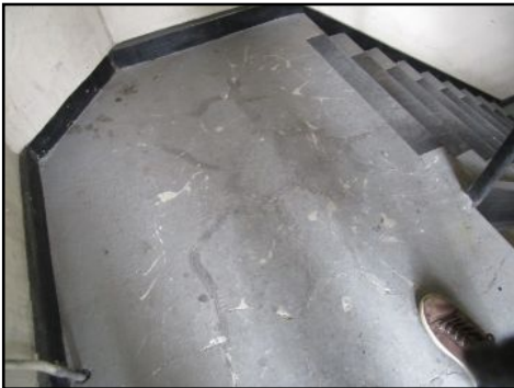
Cracked landings- needs to be serviced
