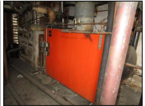
Boiler Unit was not operating at the time of the inspection for heater- we recommend that a licensed plumber evaluate the unit
