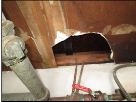
Holes in walls/ceiling areas - needs to be serviced
