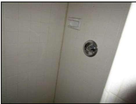
Shower pan & walks are in a worn/stained/older condition-501 - typical for the age
