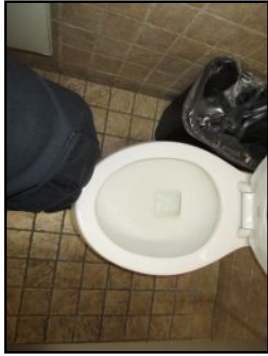
Toilet loose at floor mens 1st & 4th,5th floor & womens 1st,5th floor baths - needs to be serviced
