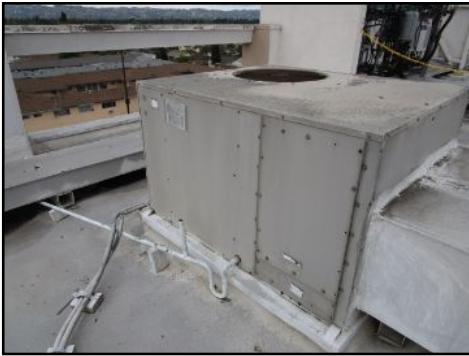
General view older unit
