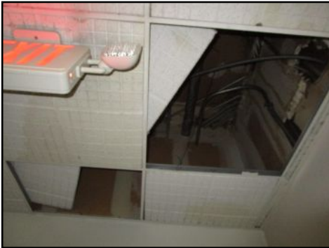
Missing loose panels 1st floor hall - needs to be serviced
