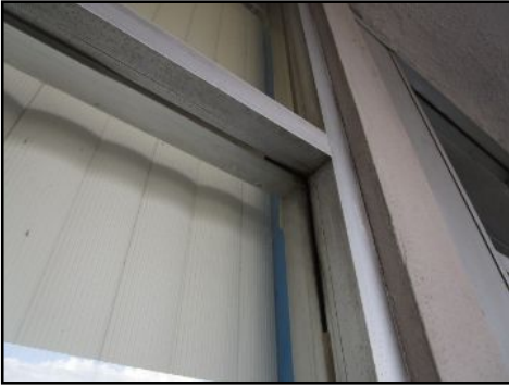
Loose/missing weather stripping
