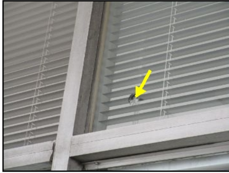
Cracked glass at rear-105,200 - needs to be serviced
