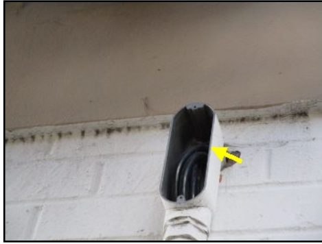
Missing j box cover at rear- needs to be serviced
