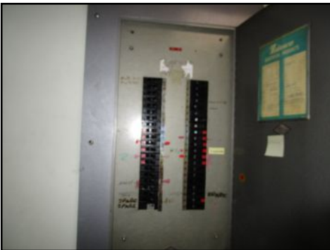
Worn/older zinsco panel present
