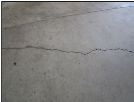
Worn with common cracks - typical for age of material
