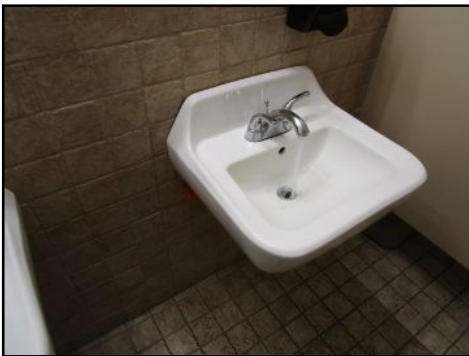
Sink Loose on wall womens 1st floors- needs minor maintenance
