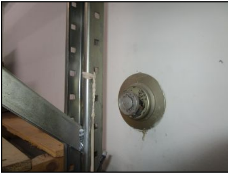
Damaged-120 - needs to be serviced
