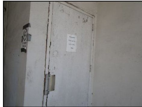
Worn/weathered at rear west side– recommend weather tight service/maintenance
