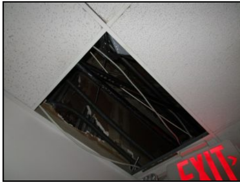
Missing loose panels 5th floor hall - needs to be serviced
