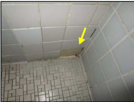
Irregular installation/patching/workmanship & missing tiles 2nd floor mens bath- needs to be serviced
