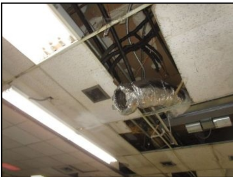
Missing register cover(s)-120 - needs to be serviced
