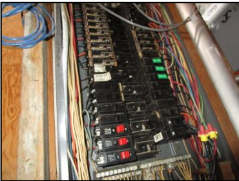
Manufacture of panel a brand (Zinsco/Federal Pacific/Stab-Lok) known for frequent issues - recommend upgrade
