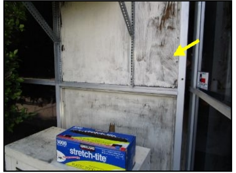
Missing glass & Windows boarded over at rear -105- consult window contractor
