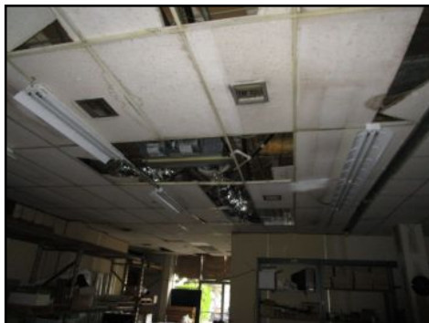
Missing loose panels -120 - needs to be serviced
