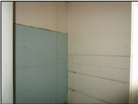
Evidence of moisture mildew smell present 2nd closet- needs to be serviced - hidden damage may exist
