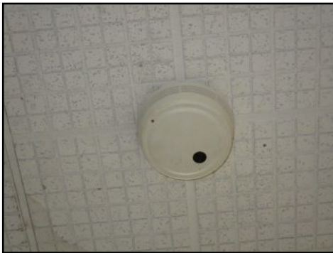
No test button - not tested
