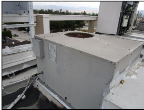
General view older unit
