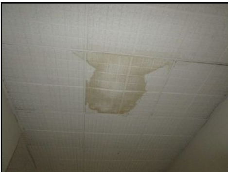
Evidence of leaking from condensation- 1st floors halls
