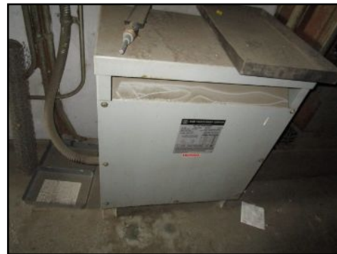
Transformer present step-down at chiller
