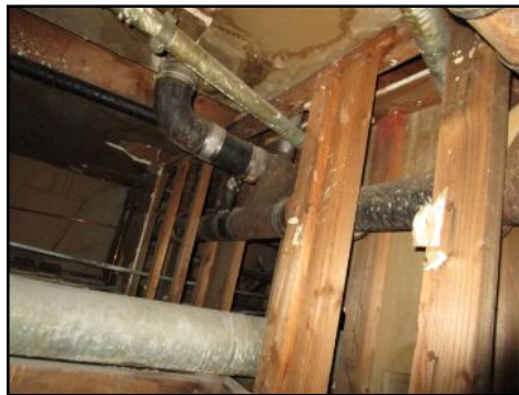
Worn/older piping system present
