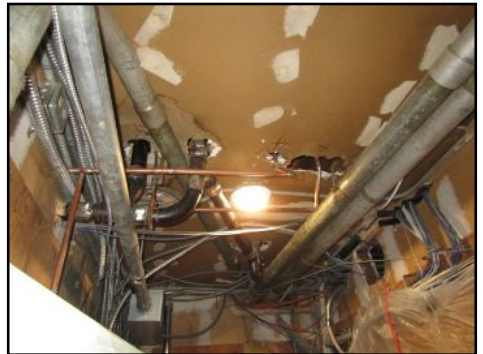
Holes large in wall 4th floor - needs to be serviced
