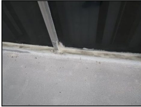
Recommend weather tight service/maintenance
