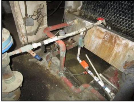
Air leak at connection to chiller uper roof- needs to be taped
