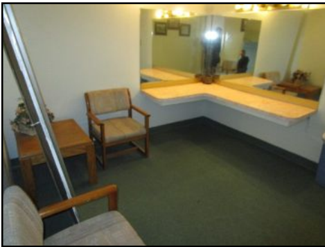
Counter is worn/scratched/older womens 2nd floor- typical wear for age
