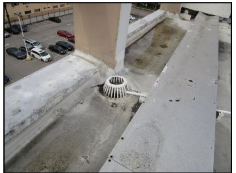
Gutters are present at the structure roof drains
