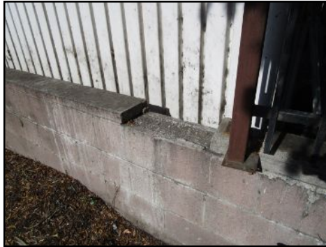
Loose areas of fencing east side- needs to be serviced
