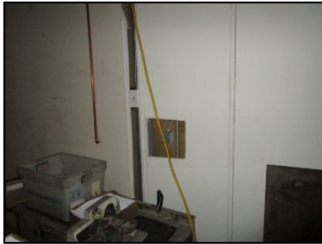
Large holes & or cracks present-120 – larger than typical - needs to be further evaluated/serviced
