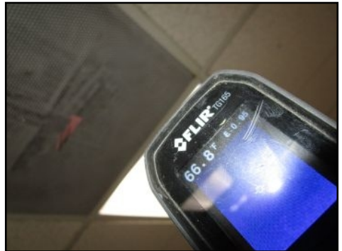
Air flow was not cold enough chiller unit-2nd floors - recommend a complete evaluation by a licensed A/C contractor
