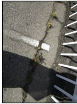
Cracking large at rear parking lot- needs to be serviced
