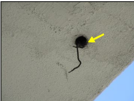
Exposed wires/connections at front over head- potential hazard needs to be serviced
