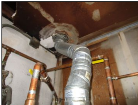
Normal wear day of the inspection - no major visible defects
