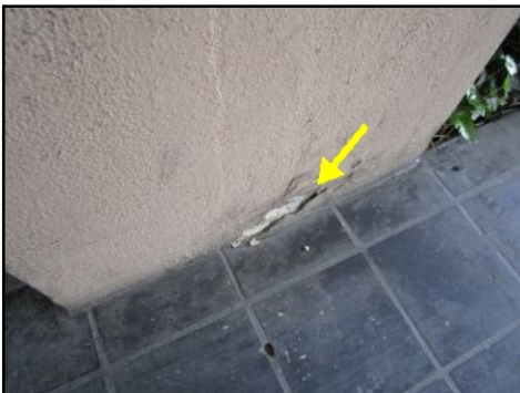
Condensation/moisture damage at front in areas- needs to be serviced
