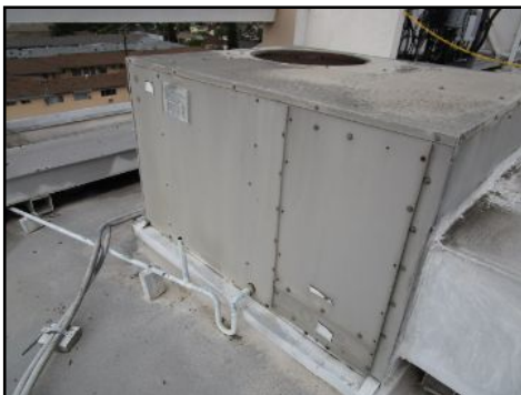
General view older unit
