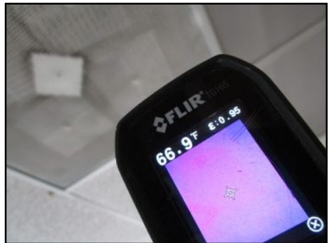
Air flow was not cold enough chiller unit 5th floors-501 - recommend a complete evaluation by a licensed A/C contractor
