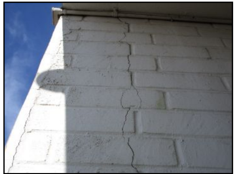
Small cracking/holes/chipping - normal for age of material
