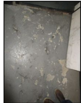
Cracked landings- needs to be serviced
