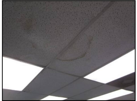
Evidence of leaking from condensation- 400
