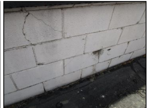
Cracking small and typical for age - monitor for further cracking and repair as needed
