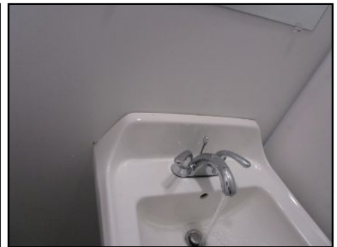
Sink Loose on wall womens 5th floors- needs minor maintenance
