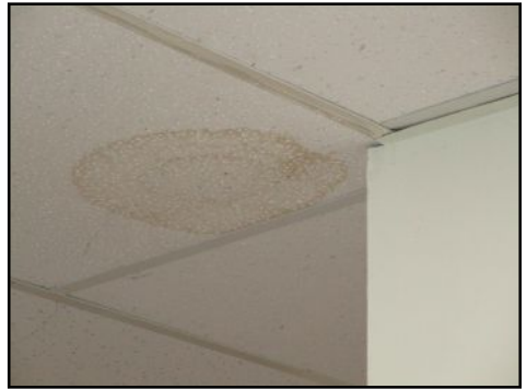
Stains/blistered areas present 300- tested dry with moisture meter
