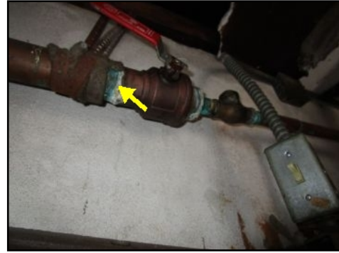
Corrosion at pipe connectors water heater - needs to be serviced
