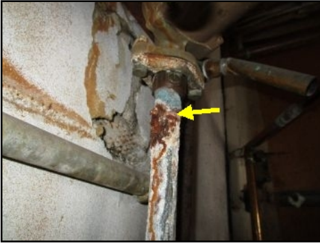
Visible leaking -water heater needs immediate attention by qualified plumber to prevent moisture related damage
