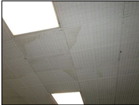
Stains/blistered areas present 1st floor hall-1st floors hall- tested dry with moisture meter
