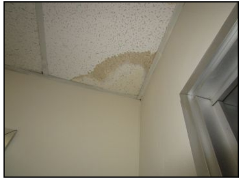
Evidence of leaking from roof-501 - needs to be serviced
