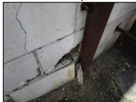
Damaged/holes block walls south side - needs to be serviced
