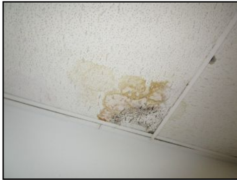
Evidence of leaking from condensation- 3rd floors halls
