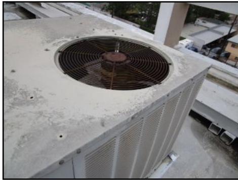
Rust visible on/in casing - needs to be serviced
