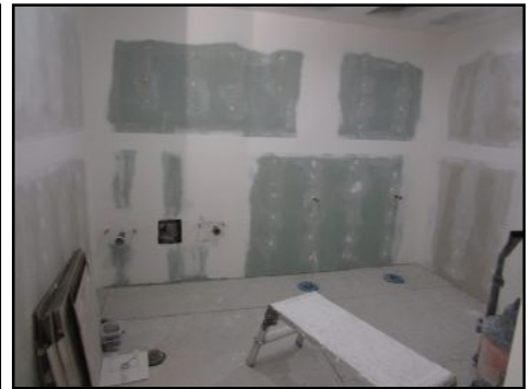
Under construction mens & womens all areas of bathroom 3rd floor - not inspected
