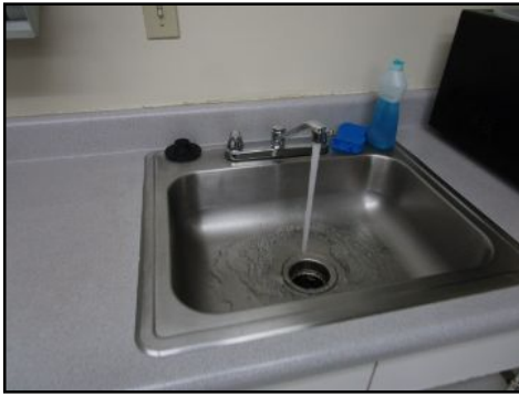
Operated at time of inspection-400
