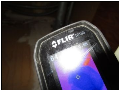
Air flow was not cold enough chiller unit- 4th floors - recommend a complete evaluation by a licensed A/C contractor
