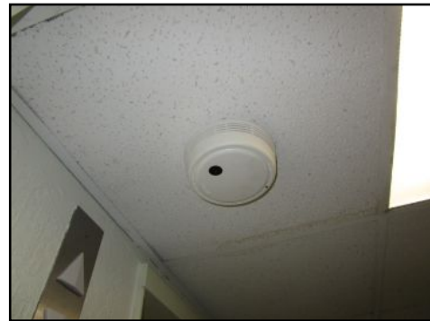
No test button - not tested
