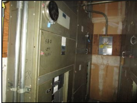
Older panel Normal wear for age at time of inspection - no major visible defects
