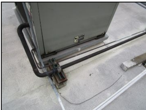
Worn/weathered insulation where visible - may need servicing/repair soon
