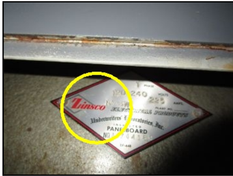
Manufacture of panel a brand (Zinsco/Federal Pacific/Stab-Lok) known for frequent issues - recommend upgrade
