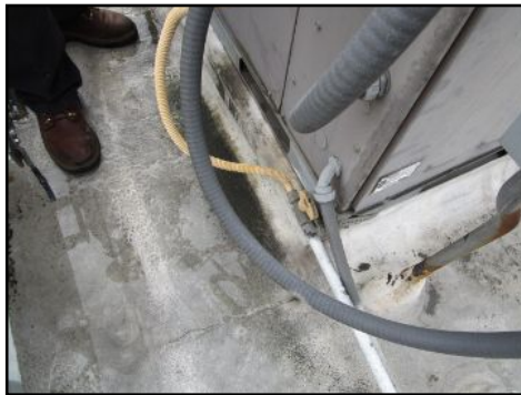
Normal wear at time of inspection - no major visible defects
