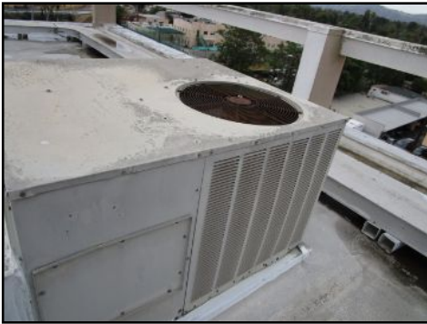
General view older unit
