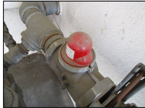
Seismic safety valve present - inspector cannot determine if valve is installed properly (seismic valves cannot be tested with this inspection)
