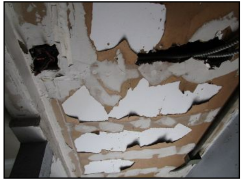
Dry water stains at chiller enclosures- unable to determine if will become active during rain
