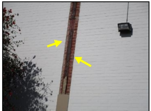
Missing in areas of the exterior at east side- recommend having a qualified contractor evaluate and repair the areas
