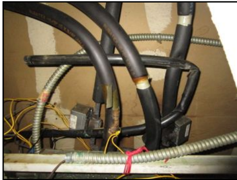
Stains present all floors - evidence of past moisture entering structure- monitor for future moisture intrusion
