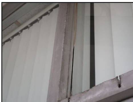
Loose/missing weather stripping
