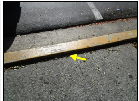
Walkway displacement/uplifted/uneven areas rear east side- potential trip hazard - needs to be serviced
