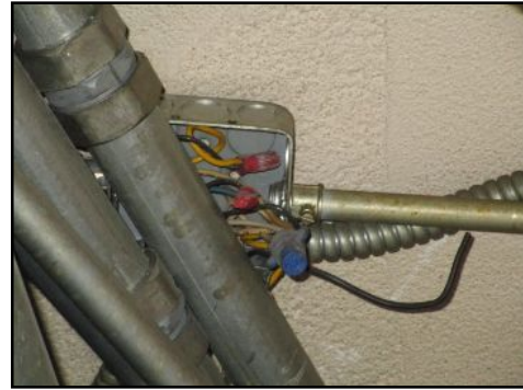
Exposed wires-501 - potential hazard needs to be serviced
