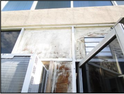
Missing glass & Windows boarded over at rear -105- consult window contractor
