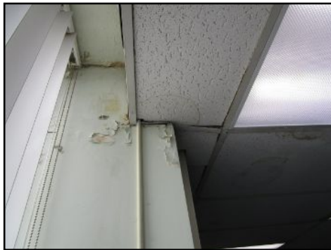
Stains/blistered areas present 400- tested dry with moisture meter at time of inspection
