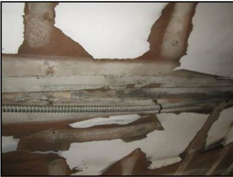
Mold like substance present upper roof -needs to be serviced
