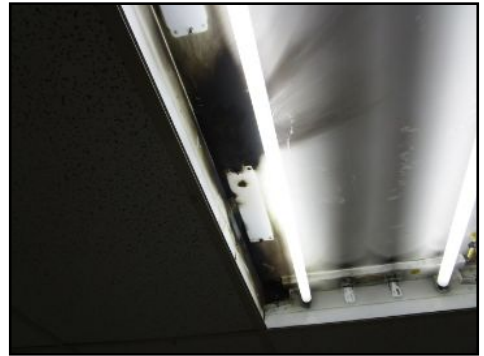
Damaged burned fixtures 400- needs to be serviced
