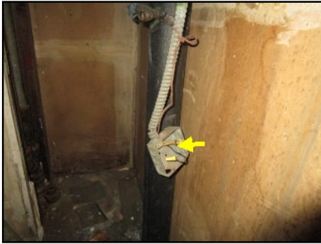
Exposed wires-120,501 - potential hazard needs to be serviced
