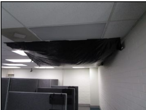
Evidence of leaking from roof-,400 - needs to be serviced
