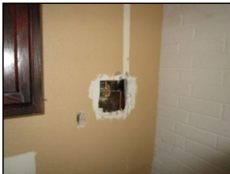
Large holes & or cracks present- 501- larger than typical - needs to be further evaluated/serviced
