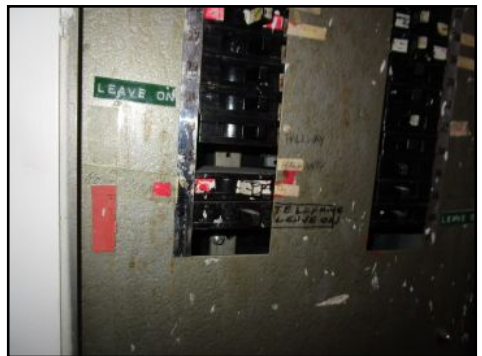
Missing knockouts/twistouts in areas - needs to be serviced
