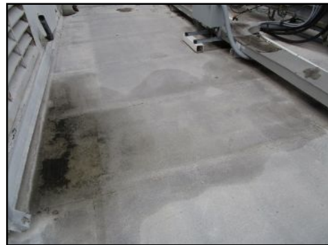
Ponding/evidence of ponding in areas - needs to be serviced
