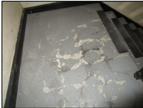
Cracked landings- needs to be serviced
