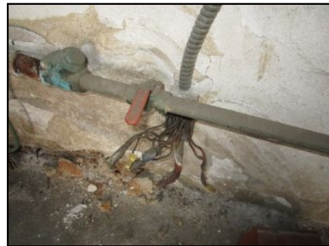
Exposed Unsecured wiring in enclosure in areas- needs to be serviced
