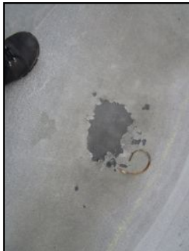
Blistered areas - needs to be serviced
