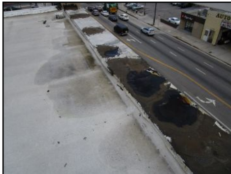
Evidence of prior repair/patching observed - consult seller for all past repairs
