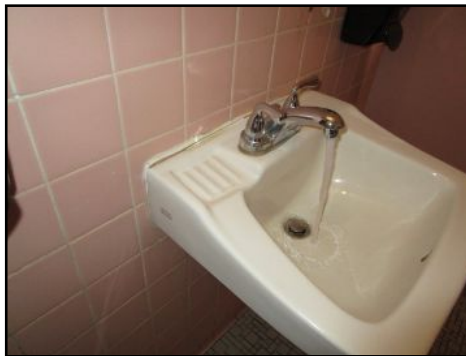
Sink Loose on wall womens 2nd floors- needs minor maintenance
