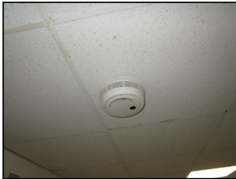
No test button - not tested
