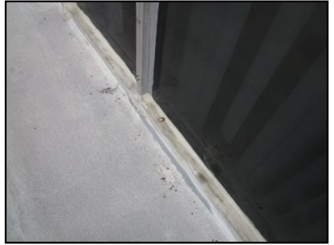
Recommend weather tight service/maintenance
