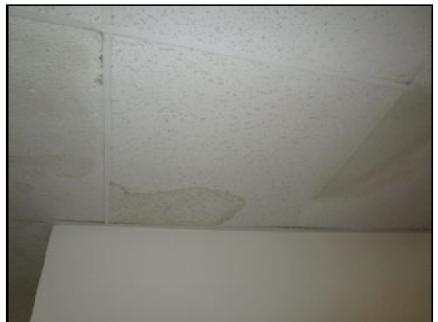
Stains/blistered areas present floors hall- tested dry with moisture meter
