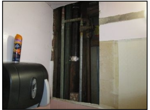
Large holes & or cracks present- 2nd floor womens bath– larger than typical - needs to be further evaluated/serviced
