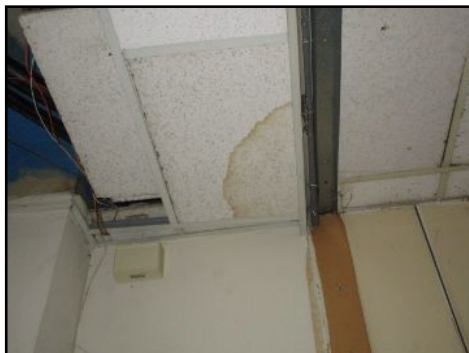
Sagging damaged materials- 120- needs to be serviced
