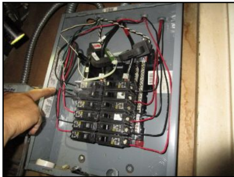
Normal wear at time of the inspection - no major visible defects
