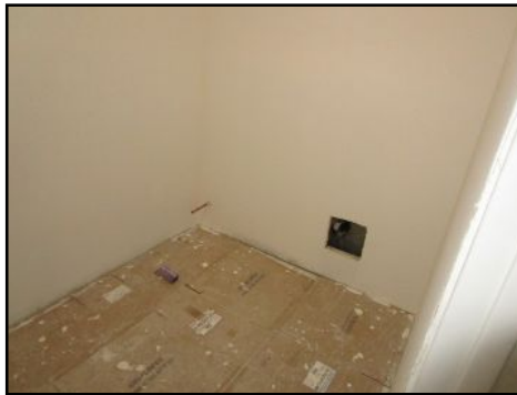
Under construction mens & womens all areas of bathroom 3rd floor - not inspected
