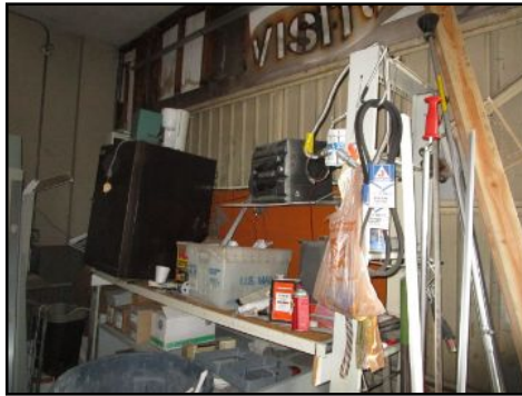
Some closet areas not visible for inspection due to personal storage
