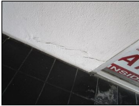
Small cracking/chipping/holes present in areas - recommend stucco service/maintenance
