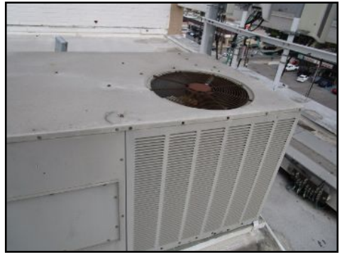
General view older unit
