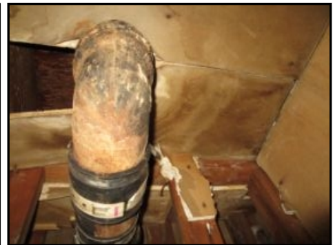
Evidence of past leakage at plumbing over bathroom 1st floor - needs to be serviced
