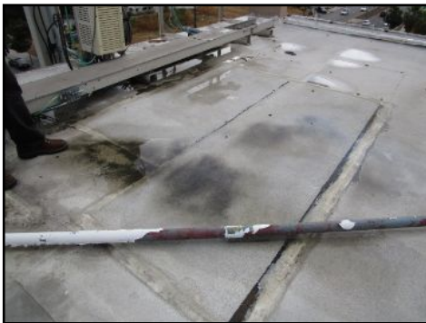
Worn and weathered materials present
