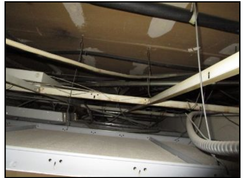
Stains present all floors - evidence of past moisture entering structure- monitor for future moisture intrusion
