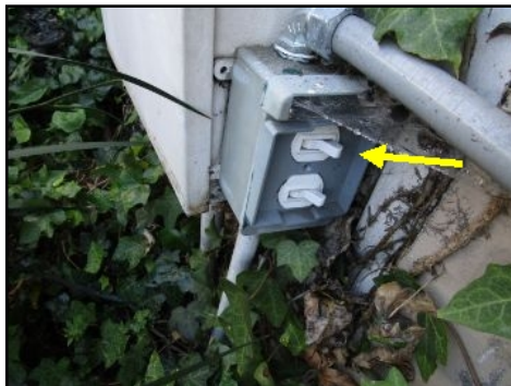
Exterior outlet/switch covers are missing or not of proper exterior weather proof type at front - needs to be serviced
