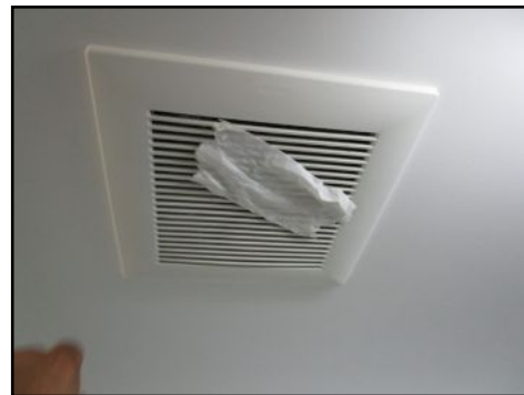
Operated at time of inspection
