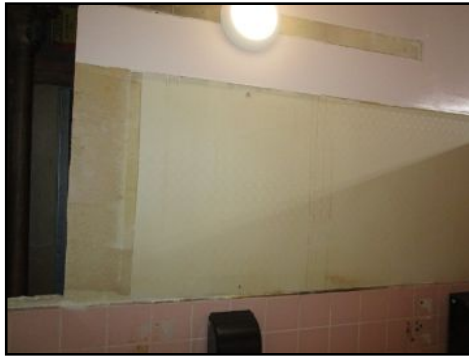
Missing mirror womens 2nd floor bath
