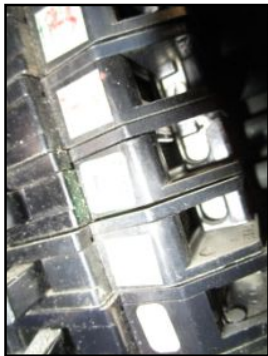
Manufacture of breakers/panel is a brand (Zinsco/Federal Pacific/Stab-Lok) known for frequent issues - recommend upgrade
