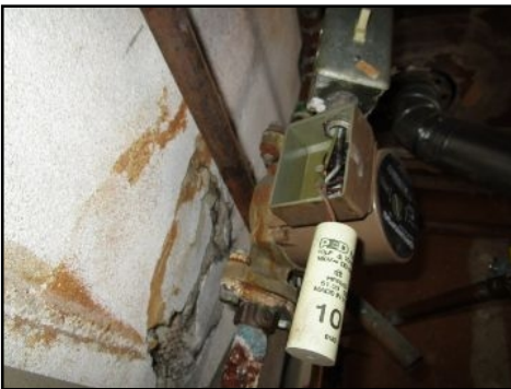
Exposed connections (splices) water pump- potential hazard needs to be serviced
