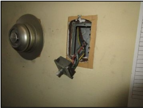
Exposed wires & connections -120 potential hazard needs to be serviced
