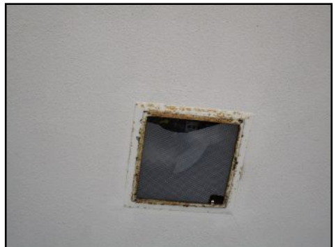
Cracked fixture(s) front over head- needs to be serviced
