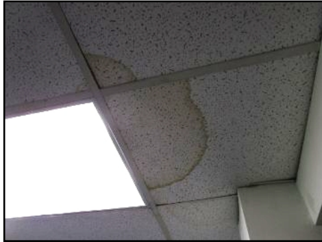
Stains/blistered areas present - ,400- tested dry with moisture meter
