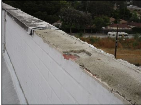
Missing/damaged flashings in areas - needs to be serviced
