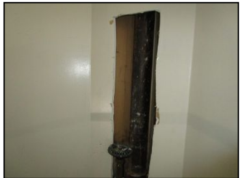
Large holes & or cracks present- in stairs walls in areas– larger than typical - needs to be further evaluated/serviced
