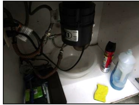
Dispose Operated at time of inspection-400
