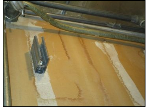
Evidence of water intrusion in the panel stained at ceiling- needs to be serviced
