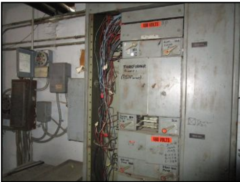
Missing covers at sub in chiller room upper roof- needs to be serviced
