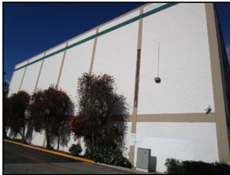
General view east side
