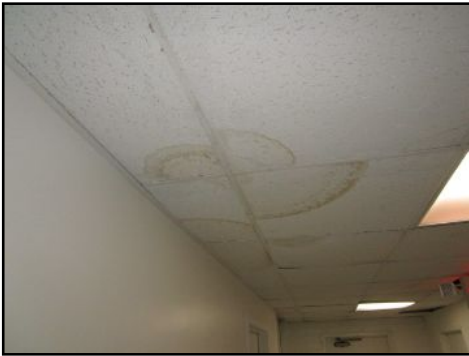
Evidence of leaking from condensation-5th floors halls
