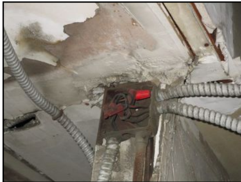
Exposed connections (splices) in enclosures- potential hazard needs to be serviced
