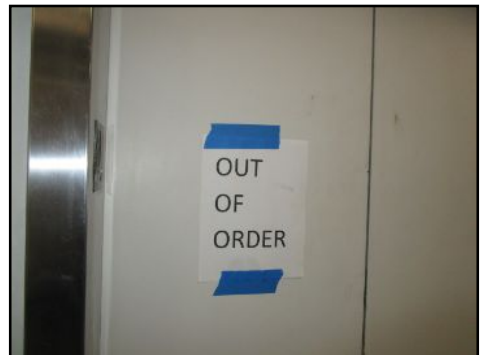
One elevator did not operate at time of inspection out of order- needs to be serviced
