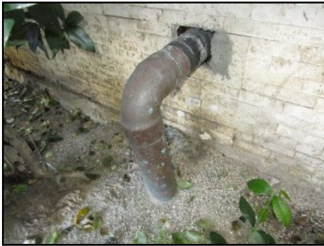
General view copper pipe
