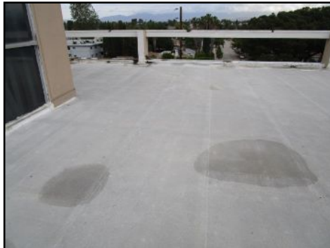
Rubber based material can hide imperfections and damaged to roof material under rubber based material
