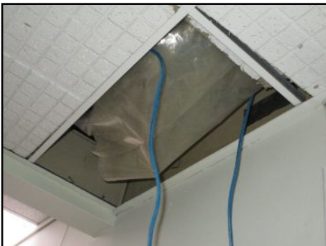
Missing loose panels 400 - needs to be serviced
