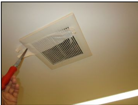
Operated at time of inspection
