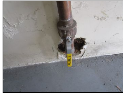
Main valve appears to have normal wear at the time of inspection - no major visible defects
