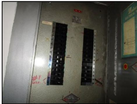
Worn/older zinsco panel present
