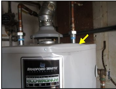
Dented areas on outer casing
