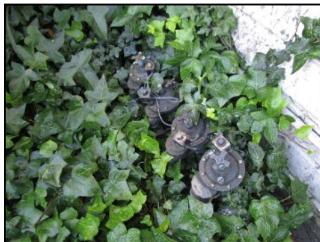
Sprinklers/irrigation systems on timers not inspected - consult seller/occupant/association/landscape contractor
