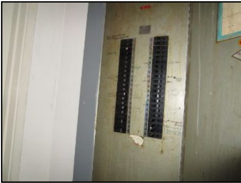
Worn/older zinsco panel present
