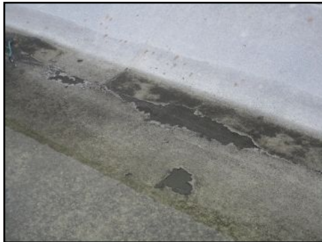
Blistered areas - needs to be serviced
