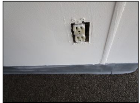
Missing outlet/switch covers - throughout structure-501 - recommend repair for safety
