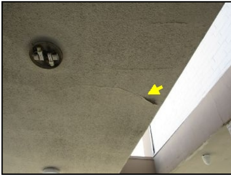
Stained & Evidence of pase leaking front & rear - needs to be serviced
