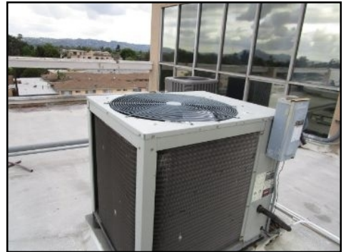
Did not operate properly two units- recommend HVAC contractor evaluate the system
