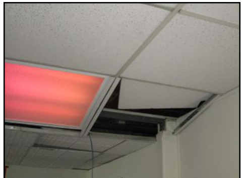
Missing loose panels 400 - needs to be serviced
