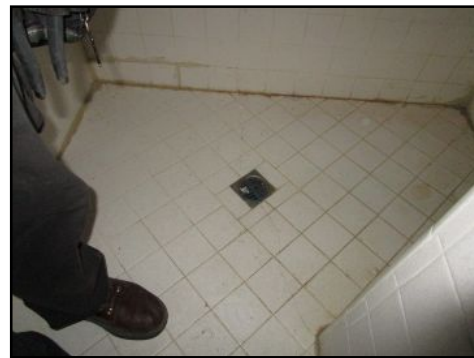
Shower pan & walks are in a worn/stained/older condition-501 - typical for the age
