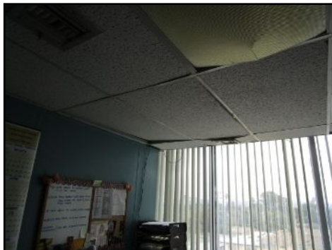
Sagging damaged materials- 400- needs to be serviced
