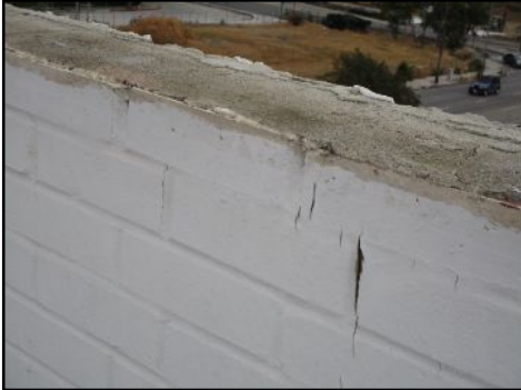
Missing/damaged flashings in areas - needs to be serviced
