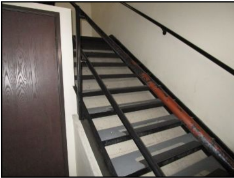
Stairs Functional at time of inspection
