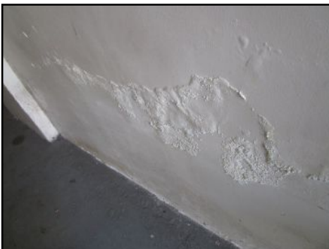
Stains/blistered areas present at hall by water main valve- tested dry with moisture meter at time of inspection
