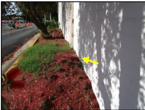
Dirt is high on east side of structure - needs to be serviced
