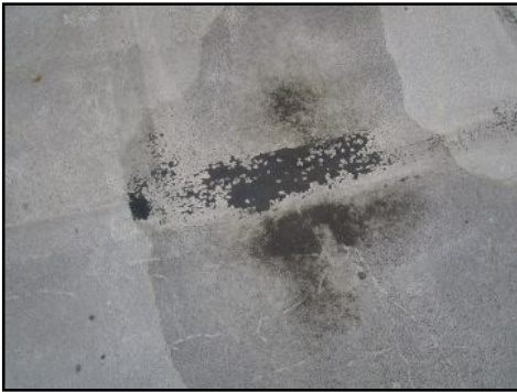
Blistered areas - needs to be serviced
