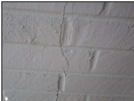
Small cracking/holes/chipping - normal for age of material
