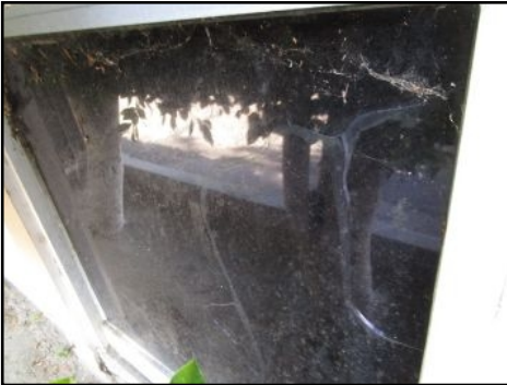
Cracked glass-105- needs to be serviced
