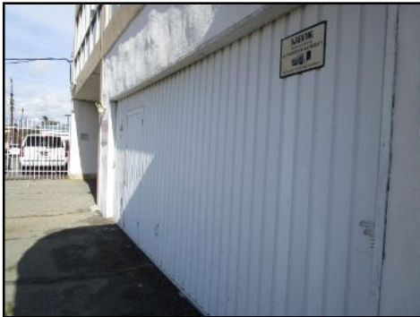
Damaged bent/dented commercial/garage doors at rear - needs to be serviced
