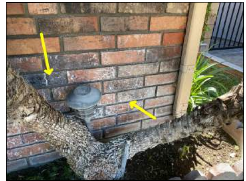
Sprinklers may be spraying side of house; check and readjust as necessary, to prevent siding damage by moisture or insects
