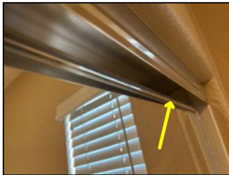
Bypass doors off tracks - needs to be serviced at southwest bedroom
