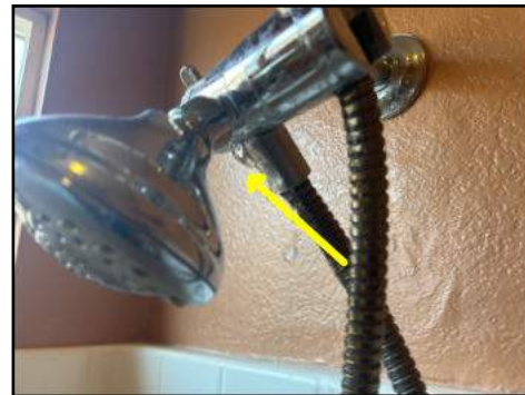
Shower head attachments leaks when operating - needs to be serviced at master
