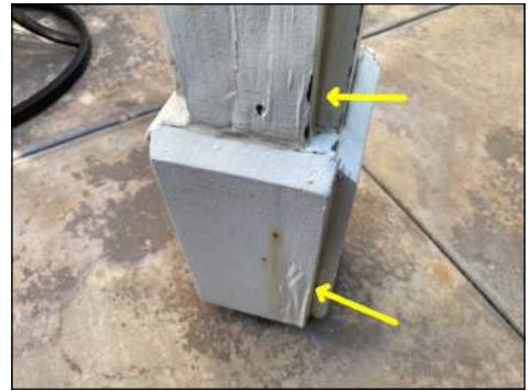
Wood deterioration observed - consult termite report
