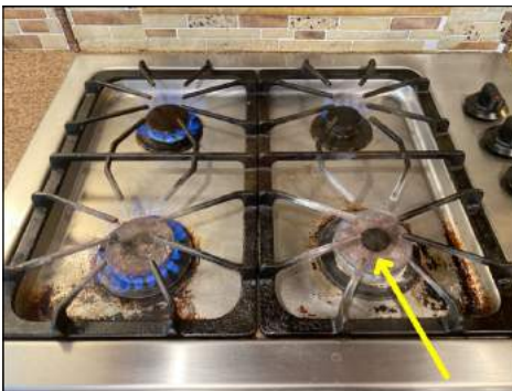
Right front element/burner not operating - needs to be serviced
