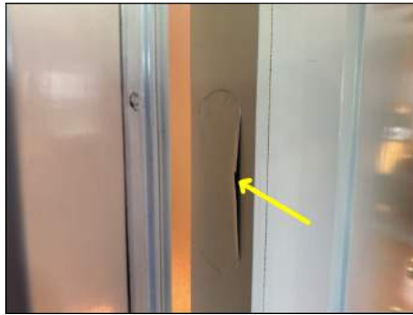
Door rating label painted over/missing - Inspector cannot determine fire rating
