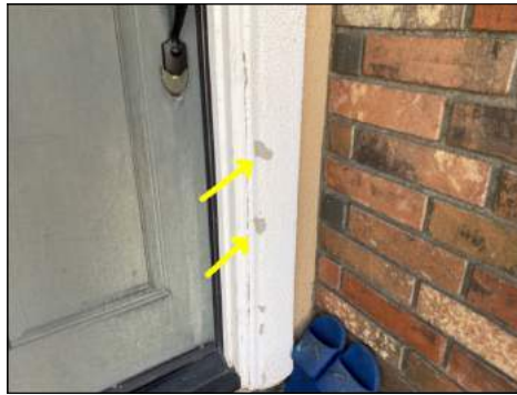
Small cracking/chipping/holes present - recommend siding service/ maintenance and sealing all holes and gaps
