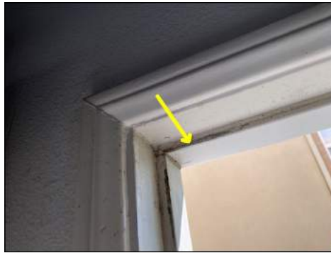
Missing weather seals at exterior door(s) - recommend servicing
