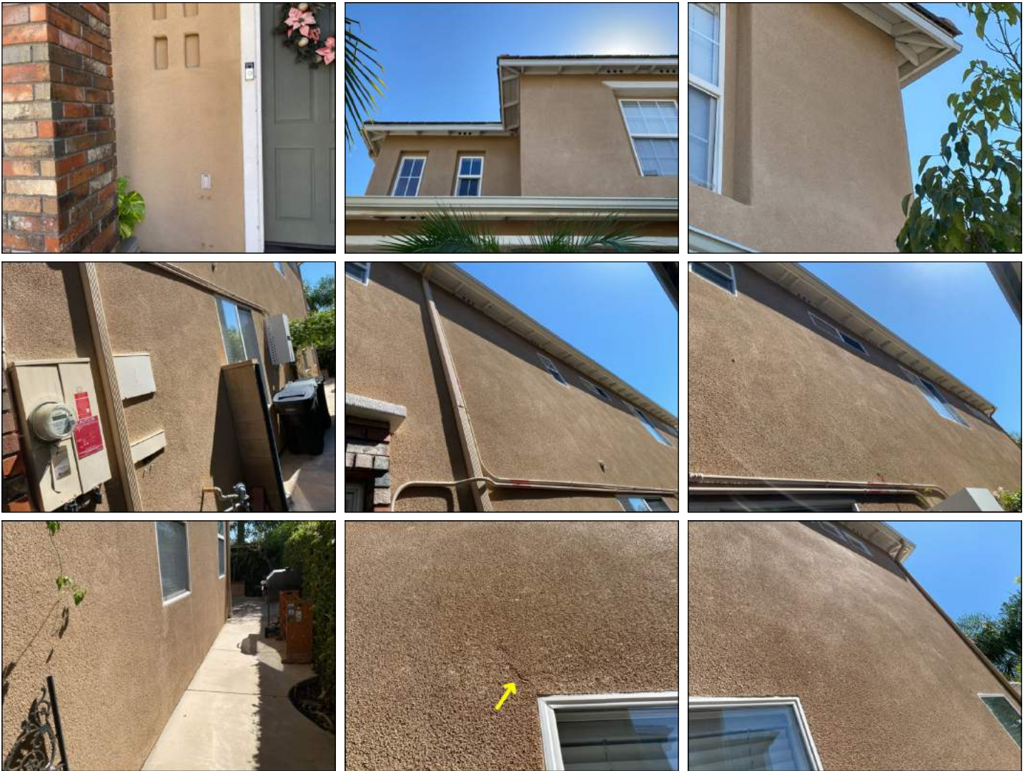
Small cracking/chipping/holes present in areas - recommend stucco service/maintenance
