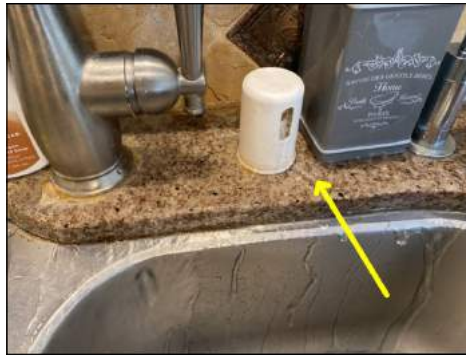
Water discharged out of air gap when draining - needs to be serviced
