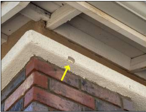
Small cracking/chipping/holes present - recommend siding service/ maintenance and sealing all holes and gaps
