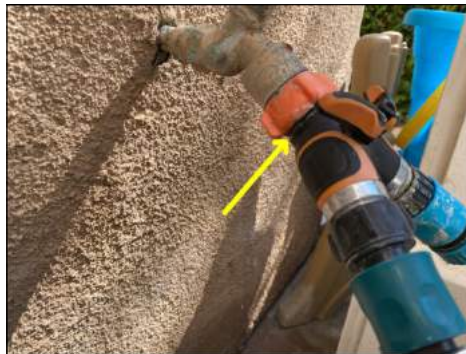
Hose bib at east side of house leaks
