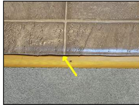
Lifting at seams - needs to be serviced - potential trip hazard
