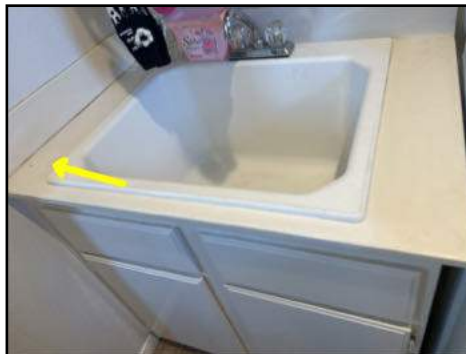
Recommend grout/sealer/stone maintenance
